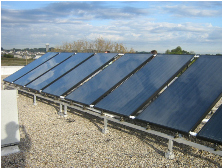
Farmer Elementary Solar Hot Water Panels
